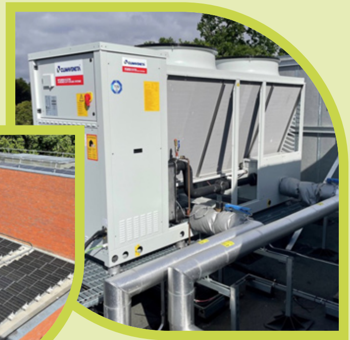
RIGHT: AIR SOURCE HEAT PUMPS INSTALLED AT CAMPUS WEST
